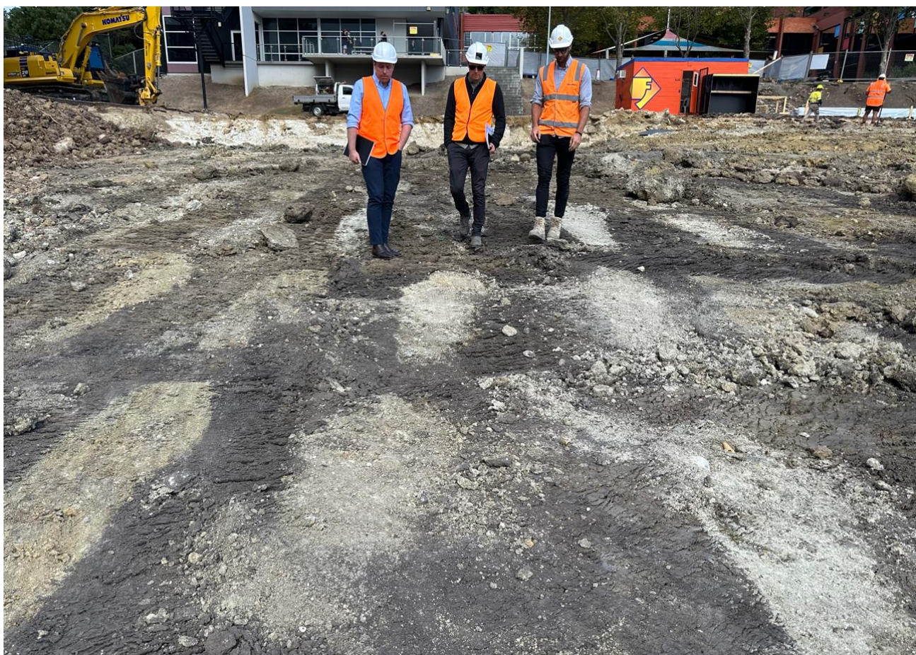
Figure 4.1.4 – Typical ground surface after bulk fill removal, showing individual burial plots.
